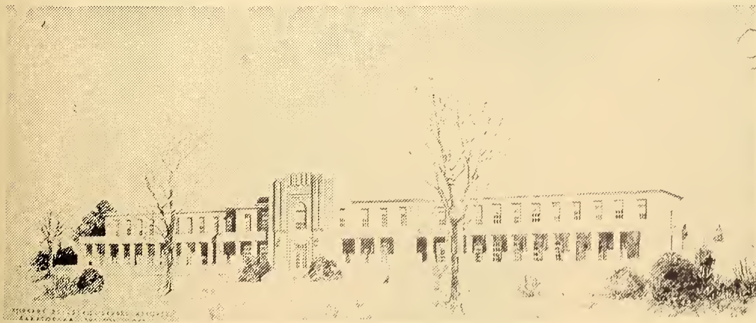
HOSPITAL BUILDING, LAUREL HEIGHTS SANATORIUM, SHELTON
